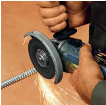
3. Cut threaded bar to exactly the required length using metal saw or right-angle grinder.
